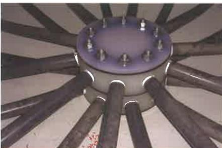
Innovative Hub Curved Underdrain follows the contour of the lower tank head to provide uniform distribution, and eliminate stagnant water hideout below. all without the need to install a concrete sub-fill.
