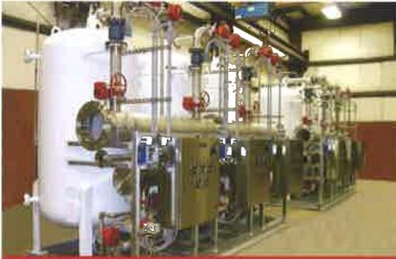
High efficiency upflow regenerated Packed Bed nitrate removal systems minimize waste and regenerant consumption
