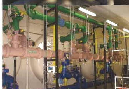
Space Saver horizontally oriented filters treat high service flows and minimize building space by locating the bulk of the tankage outdoors
